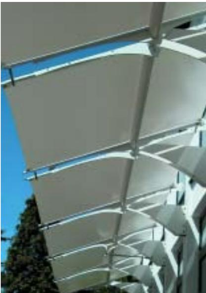
This type of system is extremely lightweight which allows large spans to be constructed without the need for additional supporting framework.
