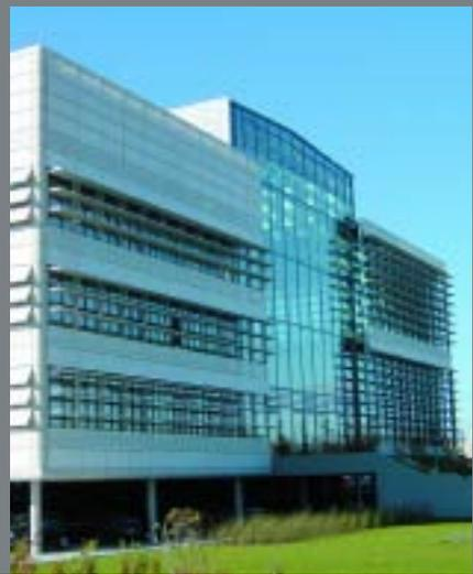
“The Colt Shadotex system allows good external vision with excellent solar protection”
